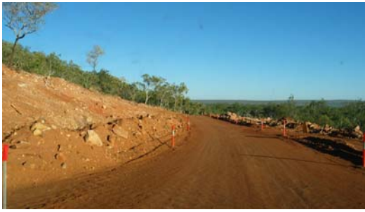
Plate 9: Structural road work
