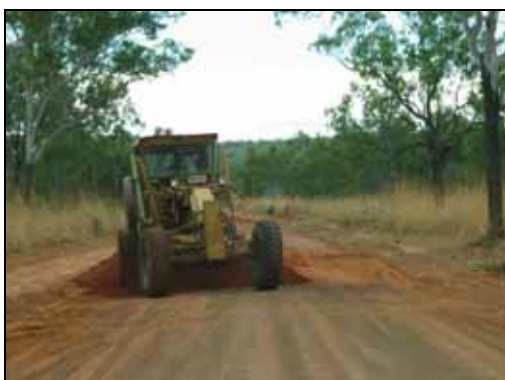
Plate 4. Grading of the GRR in progress
