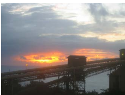
Phosphate mine conveyors at sunset
