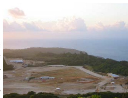
The new IRPC Site being constructed
